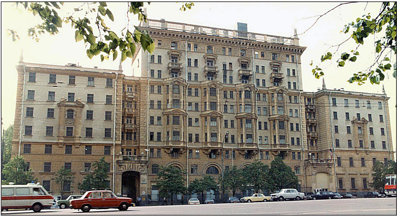
U.S. embassy in Moscow at the time of Project GUNMAN
