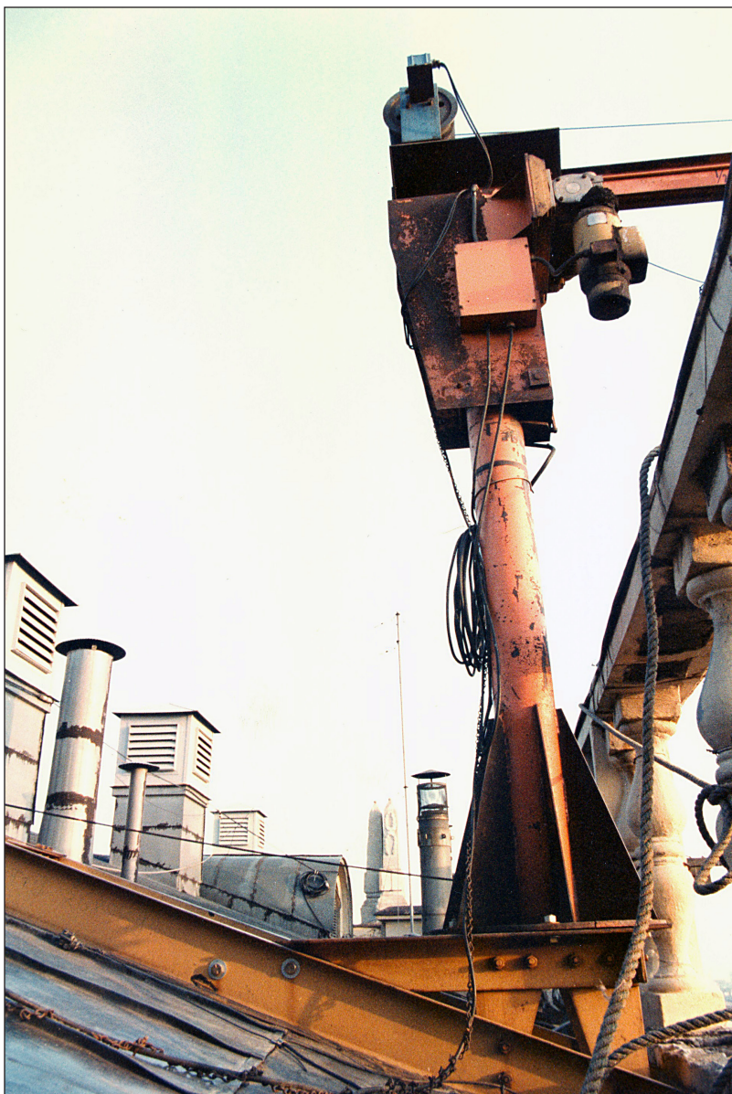
Crane winch on roof of U.S. embassy, Moscow, used to maneuver equipment
