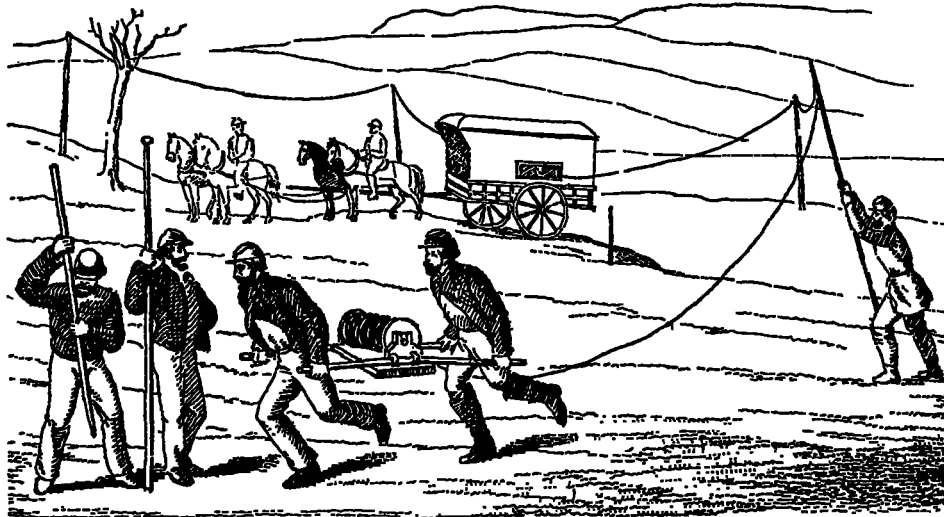
A drawing from Myer's Manual of Signals illustrating the field, or flying, telegraph. It shows the wagon with batteries and instruments. The wire (in this case presumably bare copper, since it is being strung on insulators on poles) is being run out from a reel carried by two men. The linesmen are using a crowbar to open holes to receive the lance poles. Myer estimated that 2\frac{1}{2} miles of such wire line could be put up in an hour.
